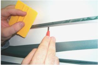
8. If any small bubbles appear during installation, they can be removed by pricking the base of the bubble with the knife blade and squeezing the trapped air out with the tip of your finger.
